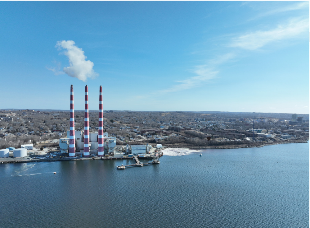
▲ Tufts Cove power generating station, located in the Narrows. During the dye release experiments and eventual alkalinity enhancement experiments, dye/alkalinity is added to the outfall pipe near the shoreline (where a bubbly white surface plume can be seen). Credit: Dalhousie University
